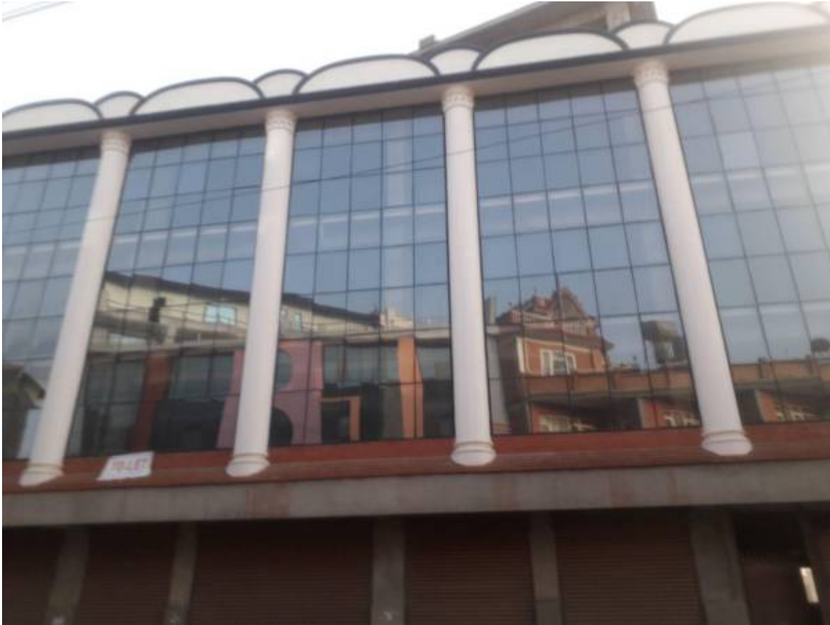
Building from the side :
