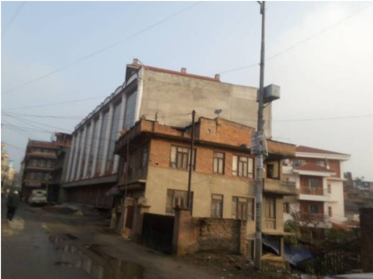
The 5ft Floor with roof access :
